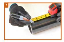
distance from the end of the pipe as indicated in the **CarbonPress®** Insertion Depth Chart.
