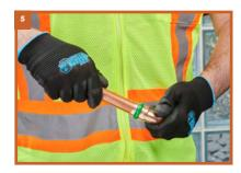
**NOTE:** if the tubing is roughly or carelessly inserted into the press fitting, it may cause damage to the sealing element.
