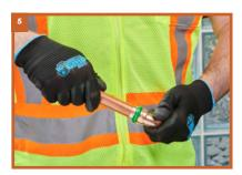
**NOTE:** if the tubing is roughly or carelessly inserted into the press fitting, it may cause damage to the sealing element.
