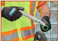
Once the jaw is removed from the fitting, the VIPR will break off, indicating a complete press.
